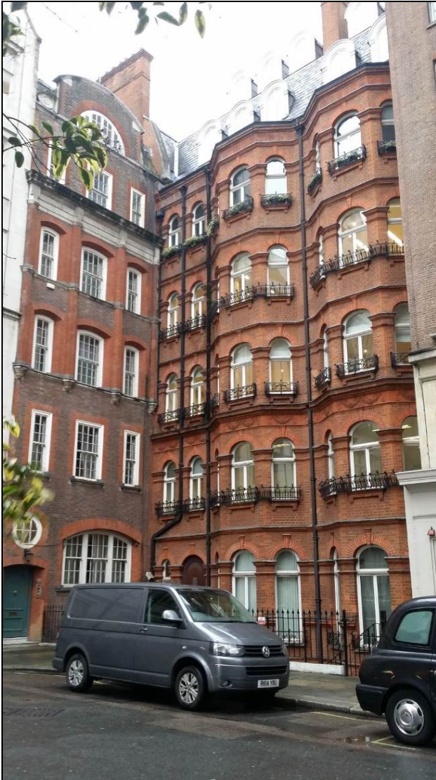
Elevation on Stratton Street
